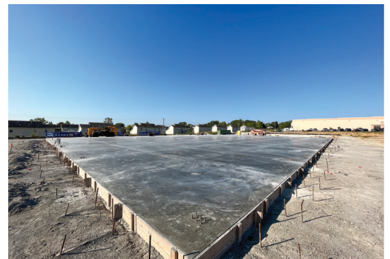
The finished slab on-grade, with curing compound, waiting for concrete strength before starting structural steel erection.
