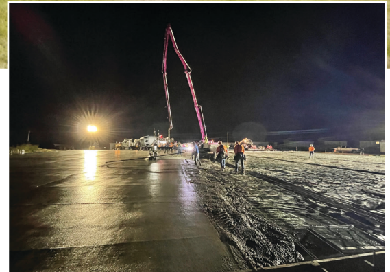
Early morning placement of the slab on grade to beat the heat for a better concrete finish.
