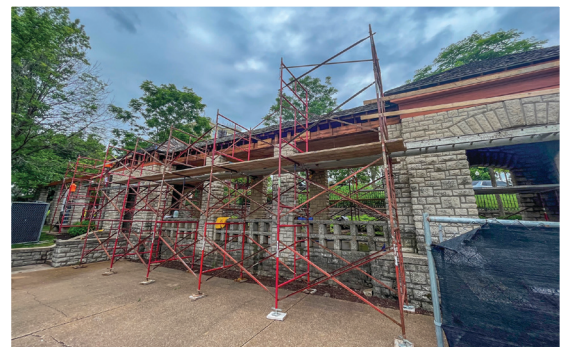
Work is underway to replace the roof and fascia.
